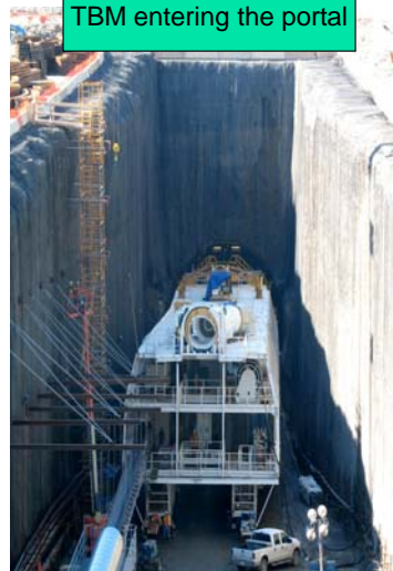
TBM entering the portal
