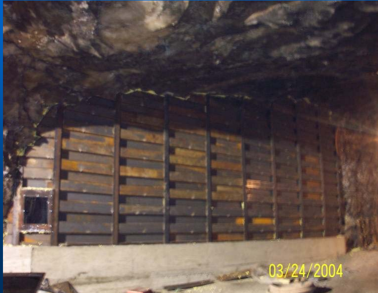
Detroit Salt Mine High Pressure air wall during construction
