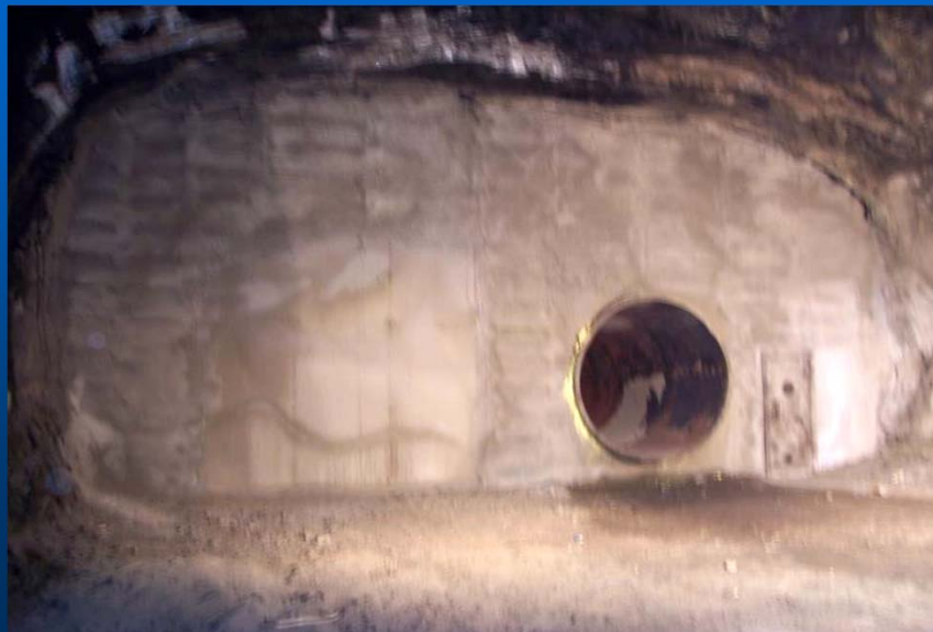
Detroit Salt Mine Completed High Pressure air wall with shot-crete
